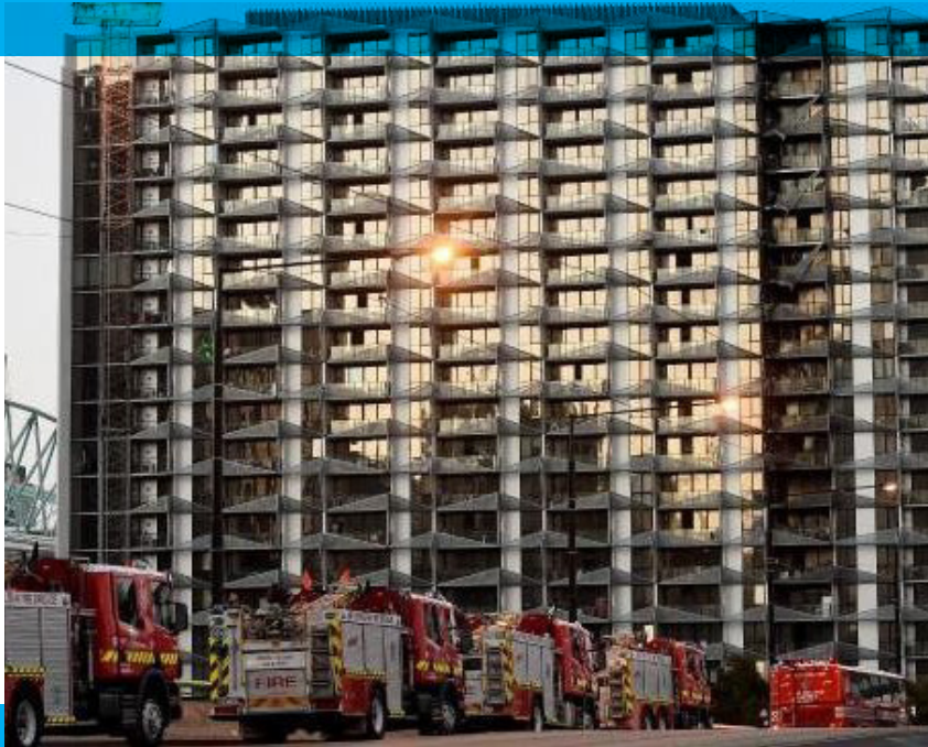
The widespread use of combustible cladding on buildings, such as Melbourne's Lacrosse Tower, led the Queensland Government to adopt new laws.
