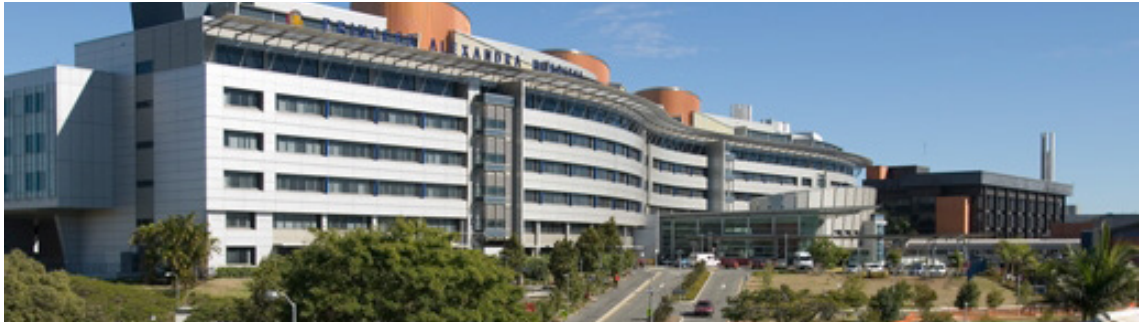
The Princess Alexandra Hospital was found to contain combustible cladding.
